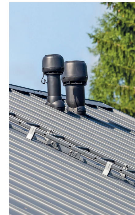
Wentylatory na dachu stromym
